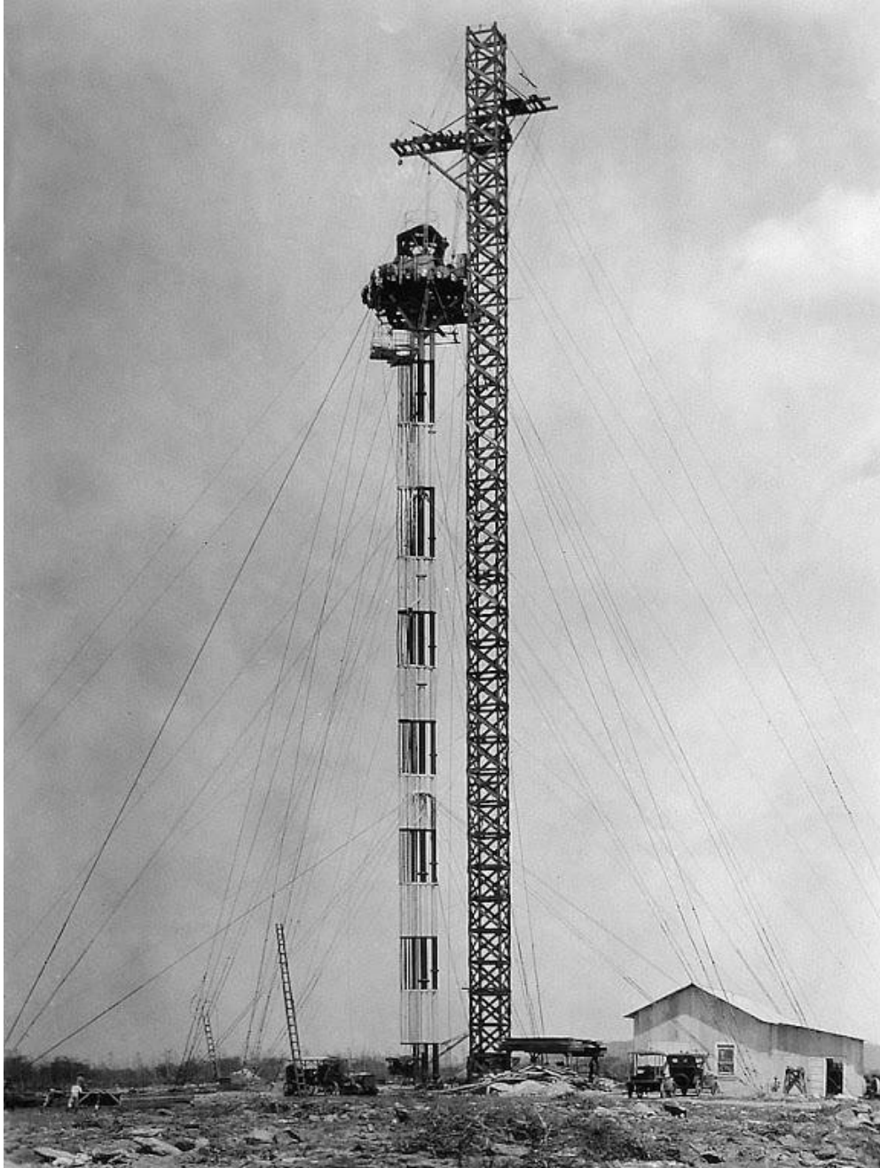
The 100-foot airship mooring mast erected in 1925 was the first aviation-related structure at Ewa.
